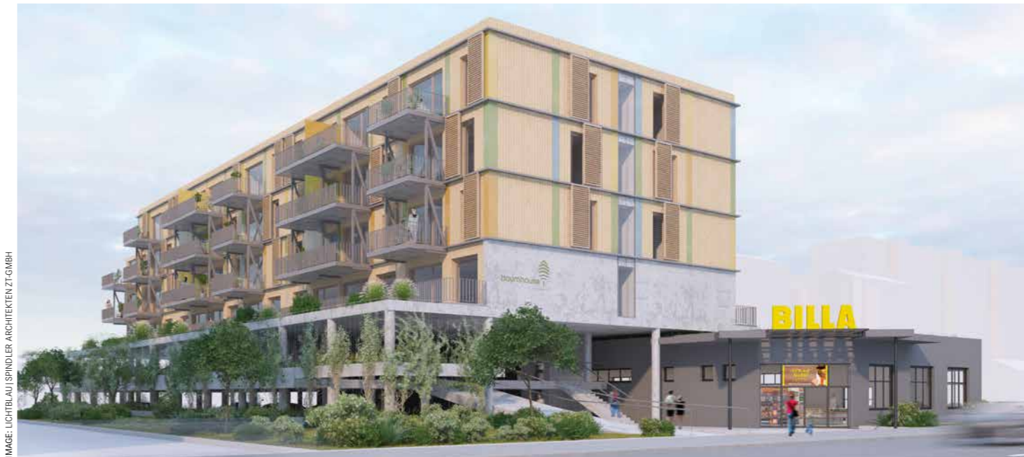
The residential building "floats" above the ground floor. The objects consist of modular timber construction for climate-neutral projects from sustainably managed forests or through steel construction.
